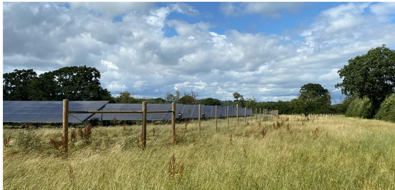
Figure 6.15: Precedent image of wooden post and wire mesh perimeter fence
